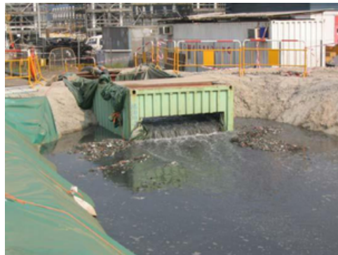
Collection of debris slurry into temporary stilling basin
